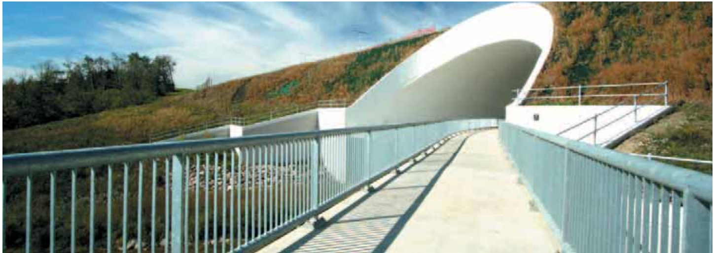
Whitemud Creek Arch Pedestrian Bridge design receives IStructE Award
