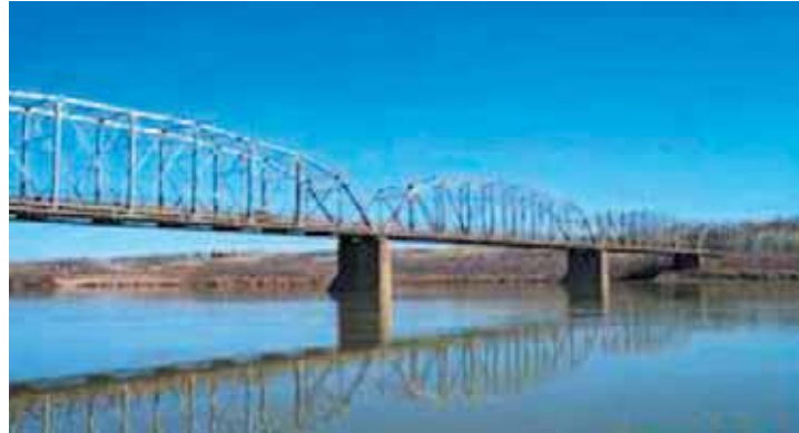
Structure on Saskatchewan Bridge Inventory
