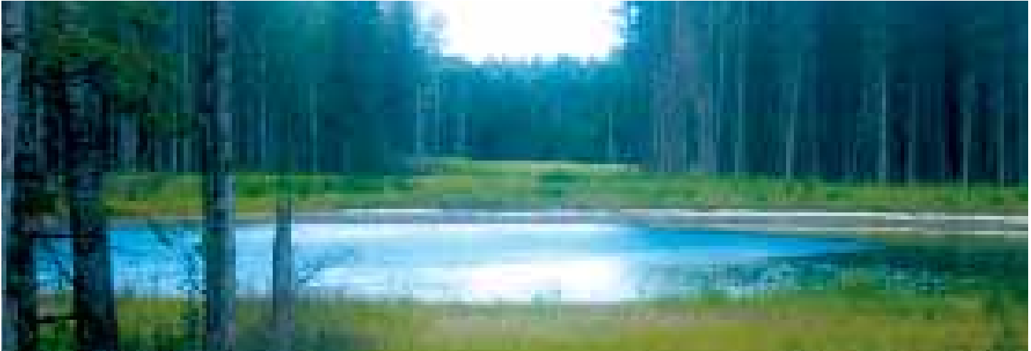
Effluent from Southshore Water Reclamation Facility is discharged to forest wetland
