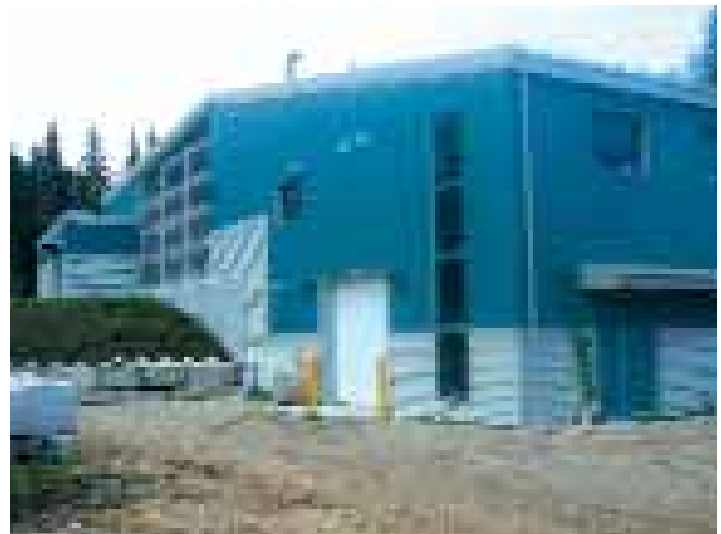
External view of Southshore Water Reclamation Facility
