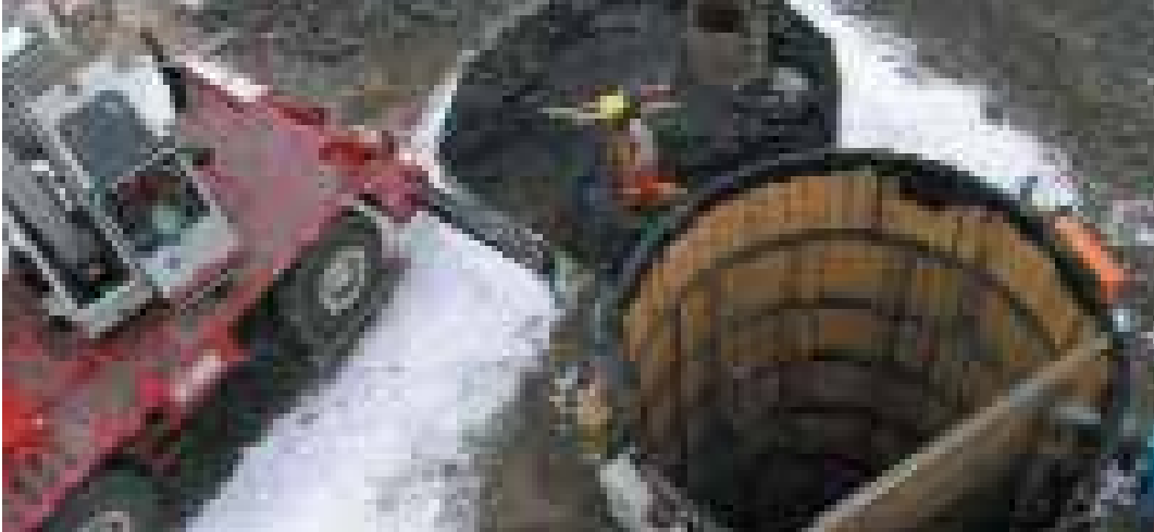
Aerial view of Dawson Park working shaft
