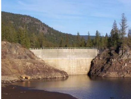
The newly expanded dam, viewed from
