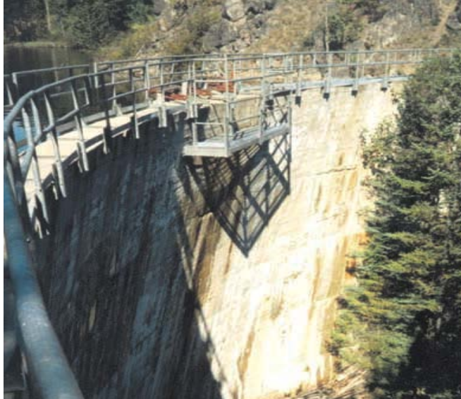
Original dam viewed from downstream.
